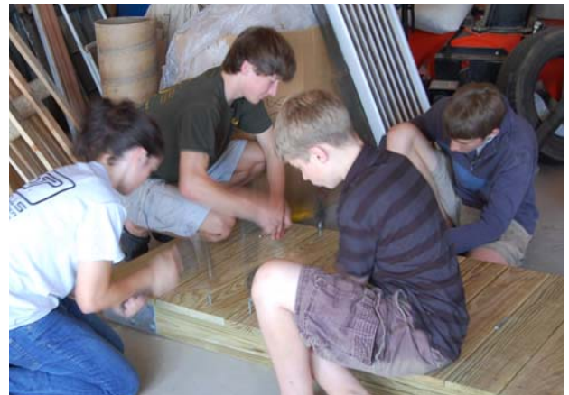
Brendan's work crew hard at work on a floating wooden dock
